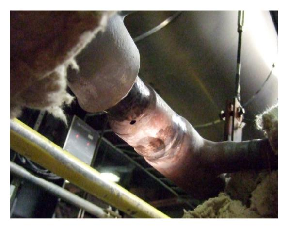
The hole in the pipe is approx 8 x 5 mm
